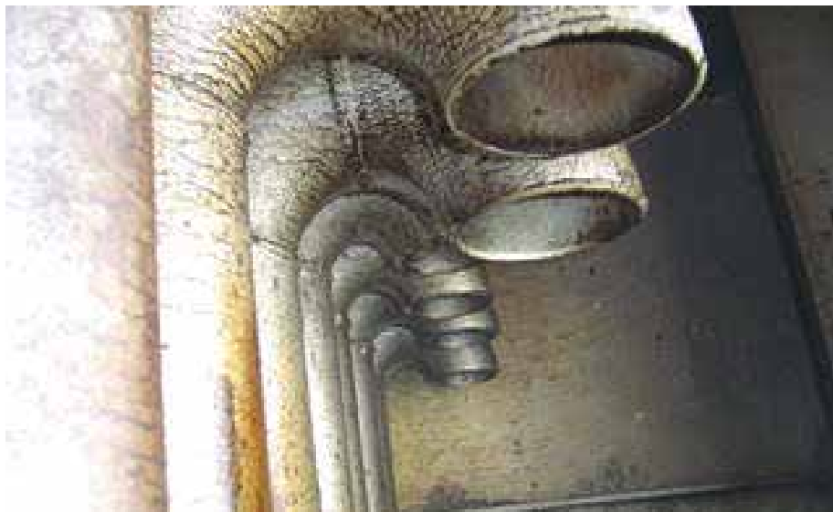
Goose neck arrangement of vent pipes inside MIST BOX
